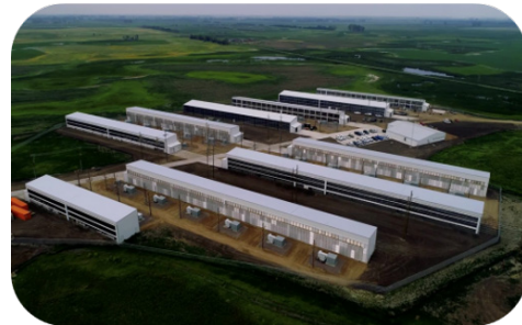
Ellendale, North Dakota Blockchain Facility 180MWs
